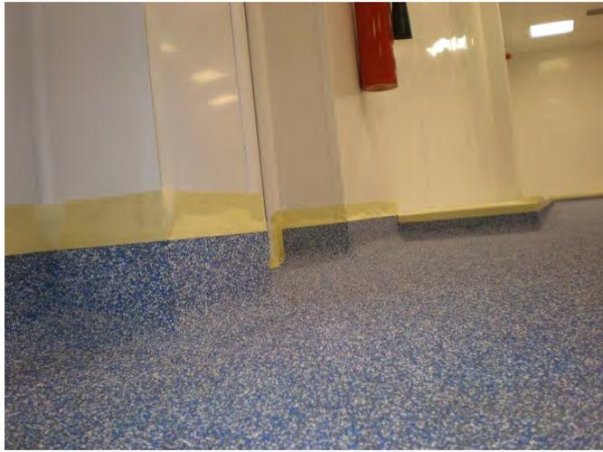
Stonclad GS mortar is used to form the cove profiles allowing a seamless transition and to facilitate cleaning. Vinyl Flakes are then applied onto the coves.
