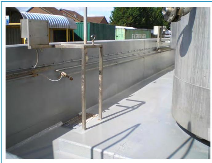
Stonclad GS mortar fillets were installed at junctions of walls/ floors to eliminate sharp corners. Stonproof crack treatment was applied to slab joints to provide strategic strengthening to the Stonchem lining system.
